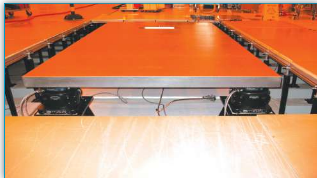
STACIS ® System on “risers” installed as a custom designed TMC Quiet Island ® subfloor platform to support an eBeam lithography tool
